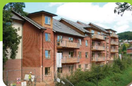
New Leadon Bank apartments
